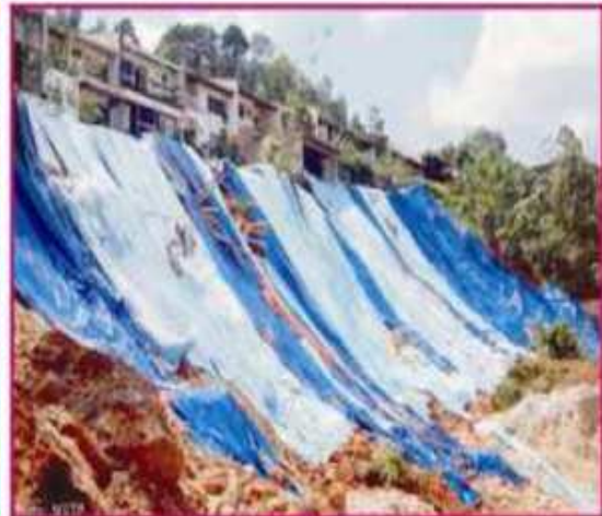
Stabilize slope material by polyethylene cover (Konkan, Maharashtra)
