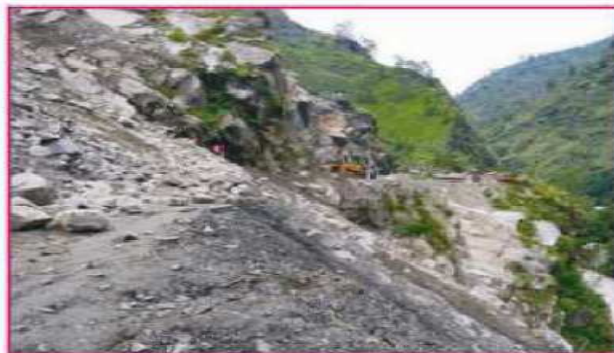
Photograph (E) landslide-on-way-to-gangotri.-preview
