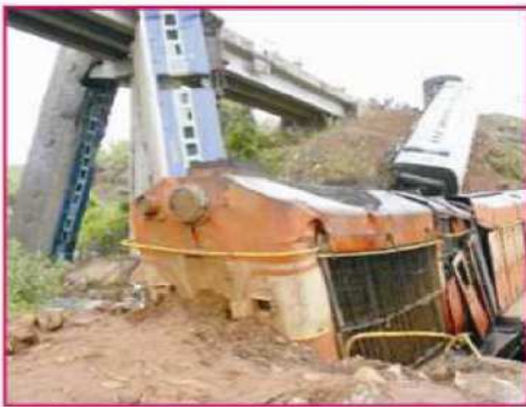
Photograph (C) Railway Bridge Collapse in Konkan Region
